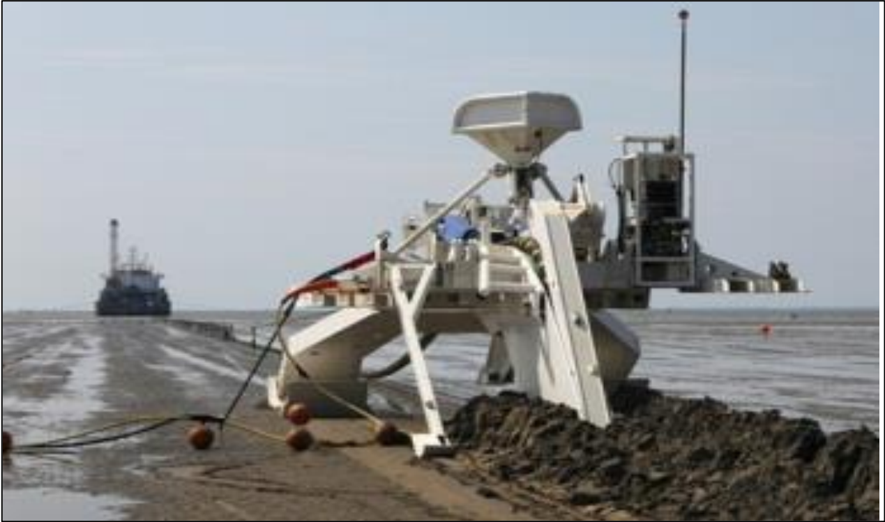
Figure 2-14: Photo showing example of an intertidal cable burial using a plough.
