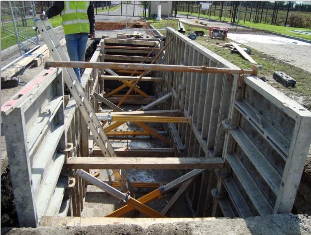
Figure 2-18: Photo showing joint bay under construction (in-situ).
