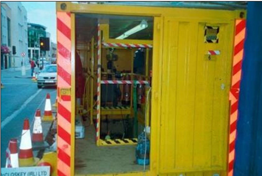
Figure 2-21: Photo of jointing container.
