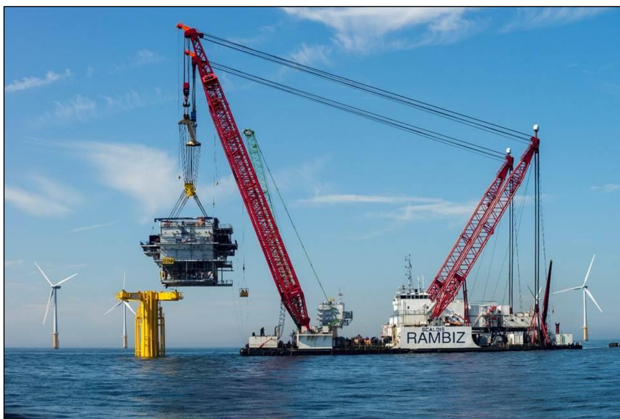
Figure 2-10: Heavy Lift Vessel installing an OSS Topside.
