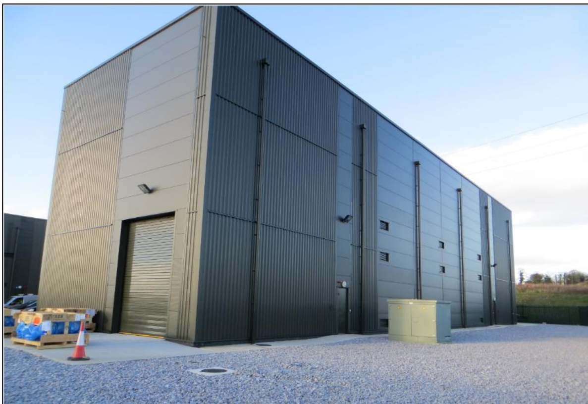
Figure 2-28: Photo of 220 kV GIS Substation Building.
