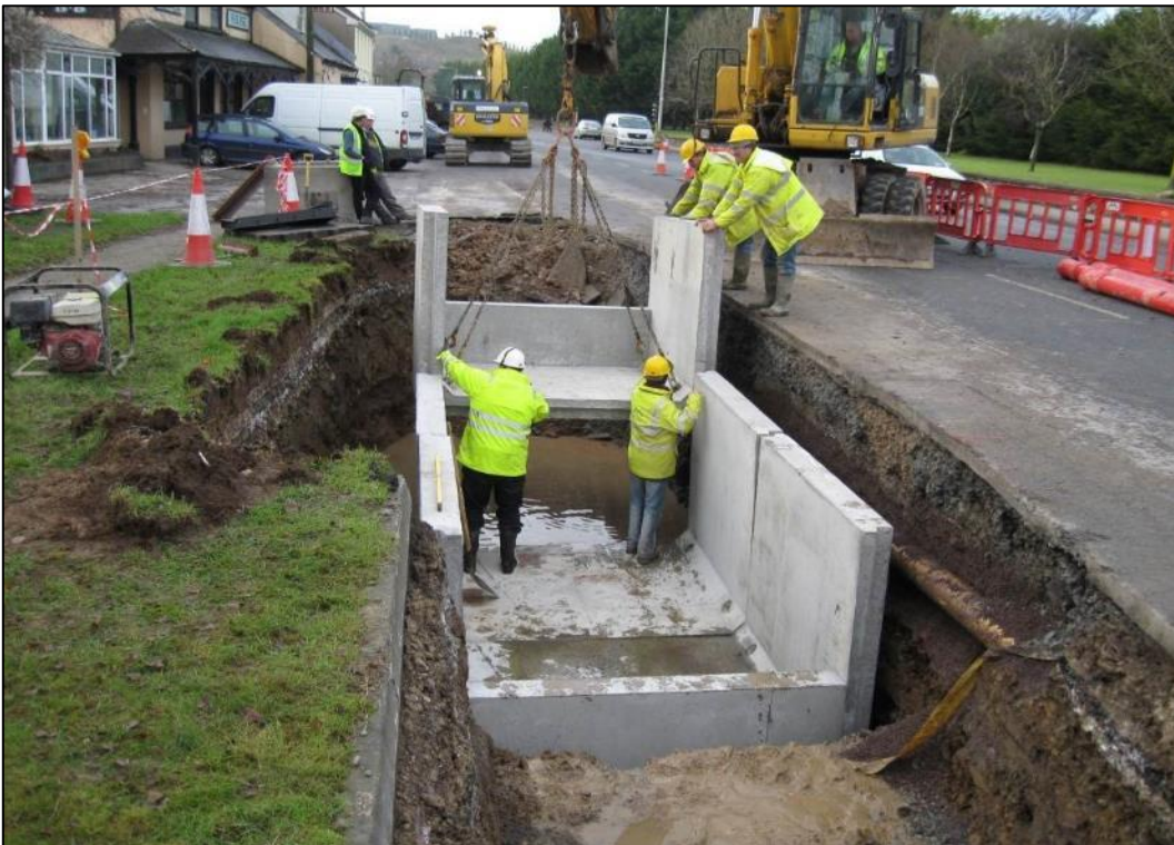
Figure 2-19: Photo showing joint bay under construction (pre-cast)
