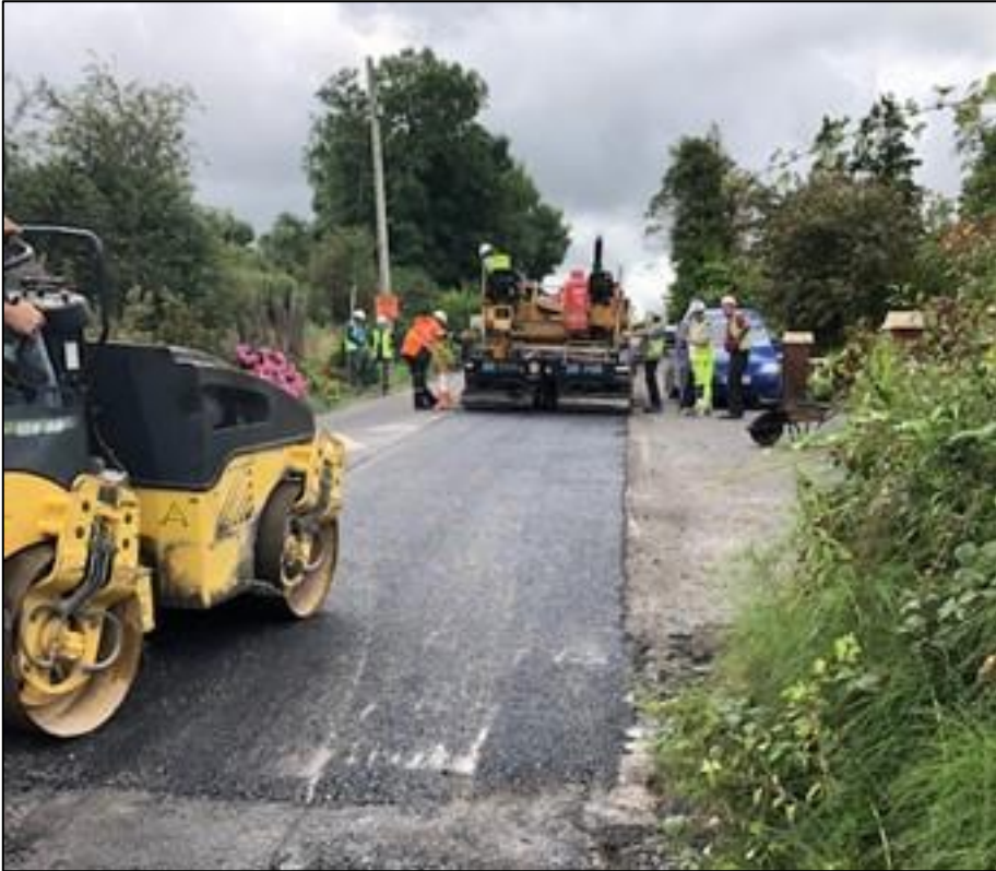
Figure 2-22: Permanent reinstatement of road surface over trench.
