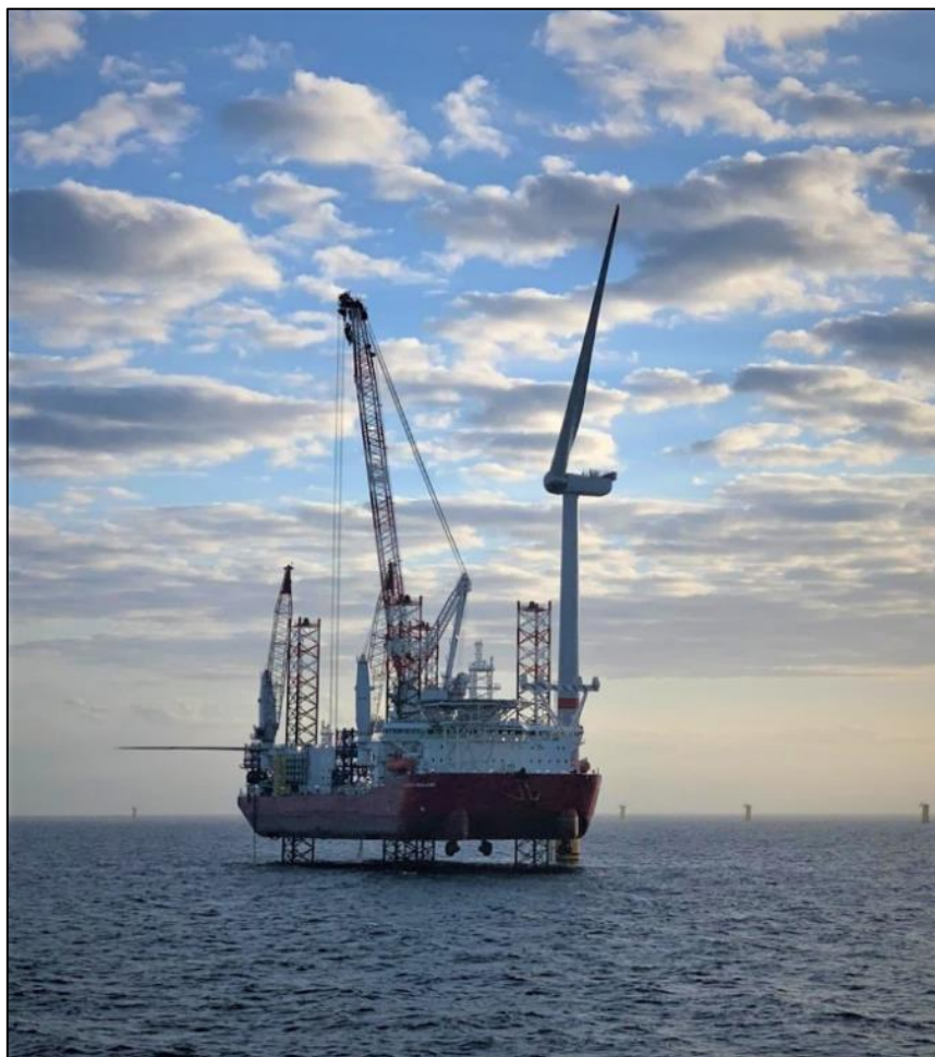
Figure 2-4: Installation vessel installing wind turbine blades.
