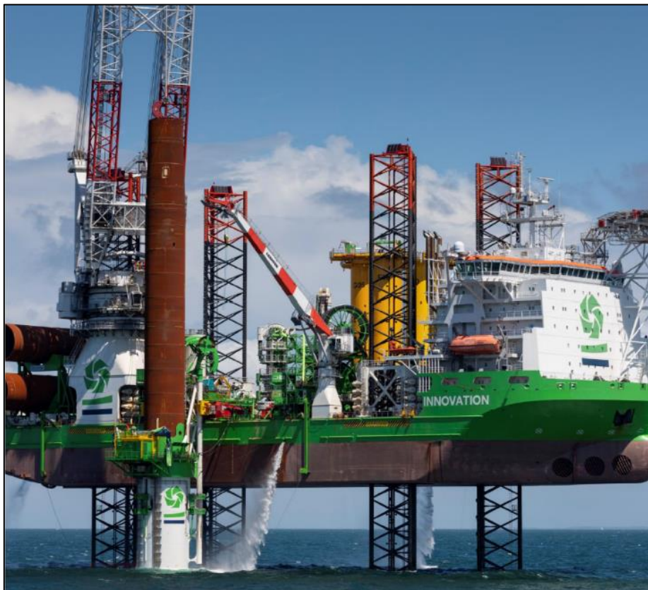
Figure 2-8: Monopile foundation installation from a JUV.
