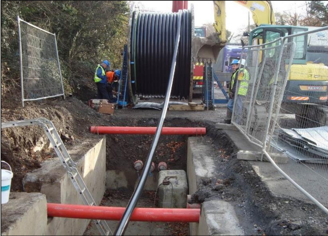
Figure 2-20: Photo of cable pulling procedure.
